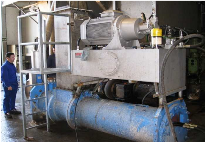
Raw material pump erected in Spain
